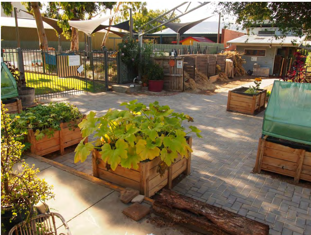
Paving completed around wicking beds:
