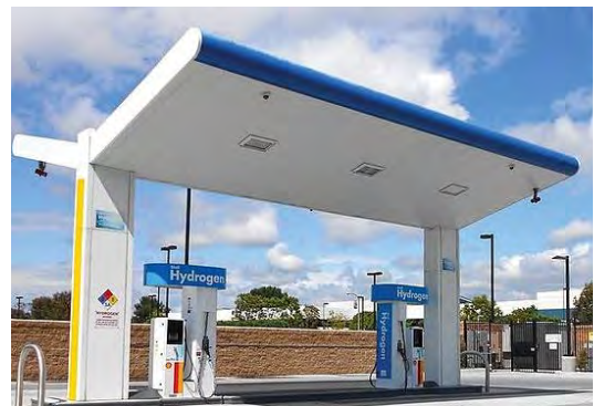
Figure 4: Hydrogen Refuelling Station
