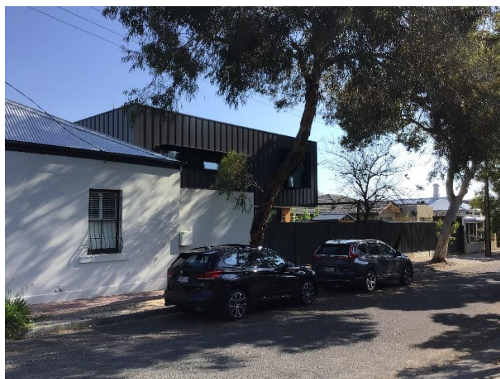
Examples of constructions built in Historic Overlay areas
