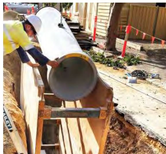
Stormwater infrastructure upgrades
