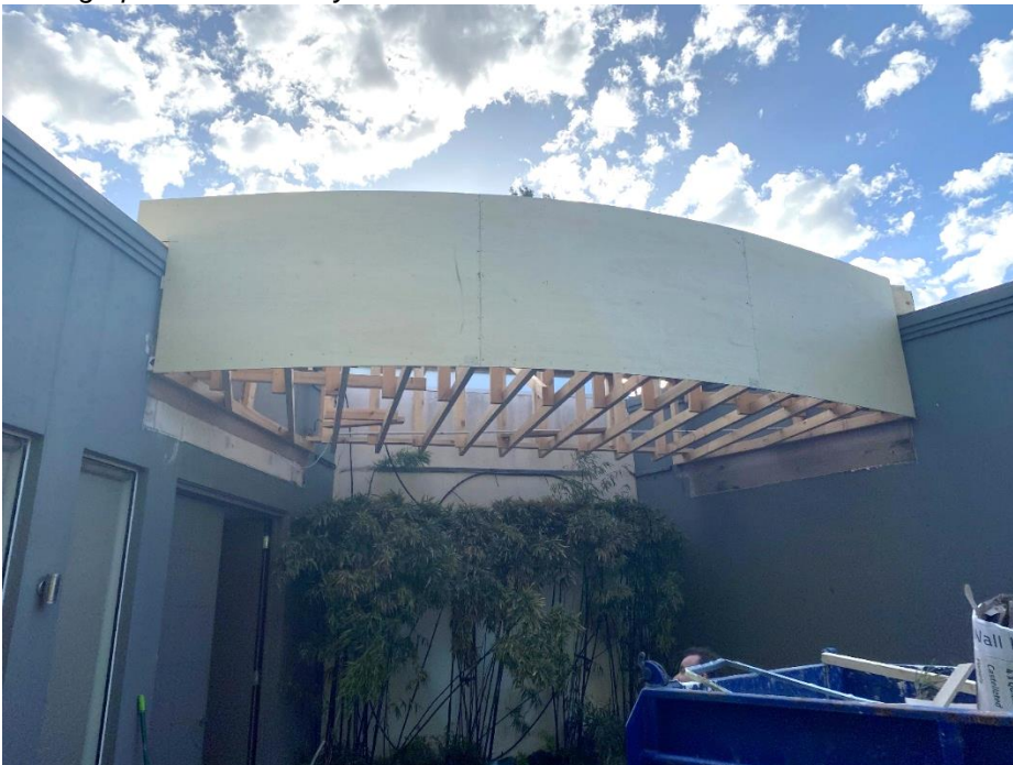
Photograph 1. Front Entry Roof
