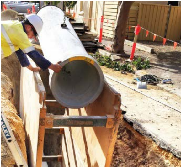
Stormwater infrastructure upgrades
