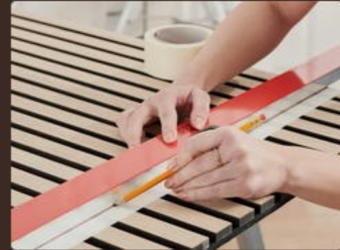
Step 2. Mark the cutting lines on the panel with a pencil and tape.
