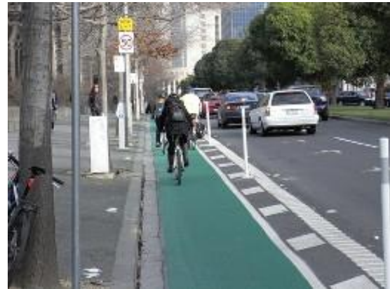
Photo 29: Separated Bicycle Lanes between the kerb and parked cars in Melbourne
