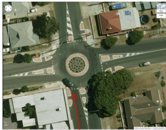
Photo 35: Radial Roundabout at Fletcher Road/Wills St, Largs Bay – slower speed (note: arrow shows direction of motor vehicle)
