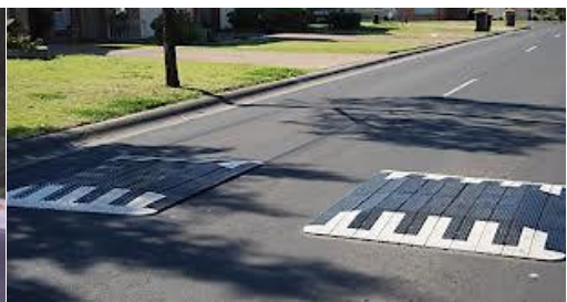
Photo 13: Speed cushions / Road humps, typical
