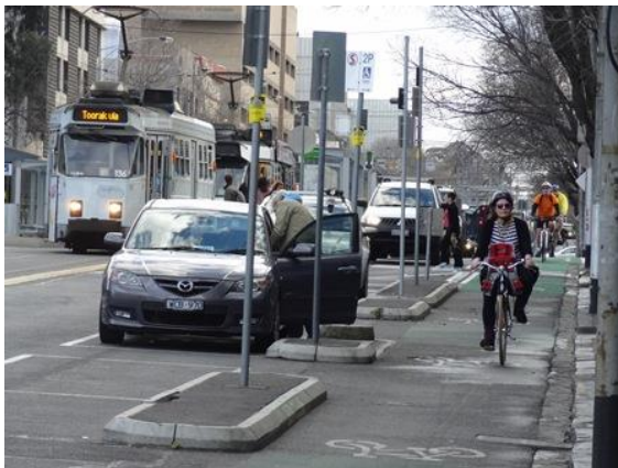
Photo 30: Kerb Separated Lane, Swanston Street Melbourne
