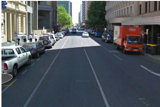
Photo 26: Pirie Street - previous narrow bicycle lanes
