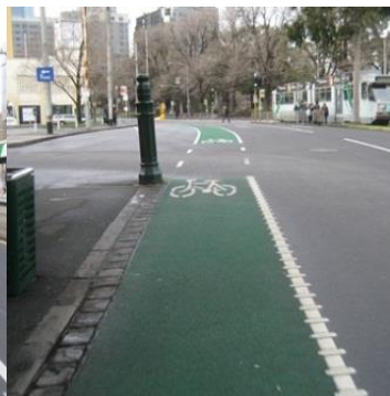
Photo 24: Tactile line-marking and green coloured lane
