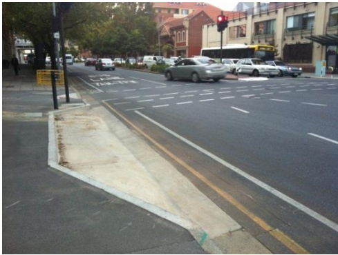
Photo 32: Cyclist Refuge for right turn at traffic signals (Grenfell Street/East Terrace, Adelaide)
