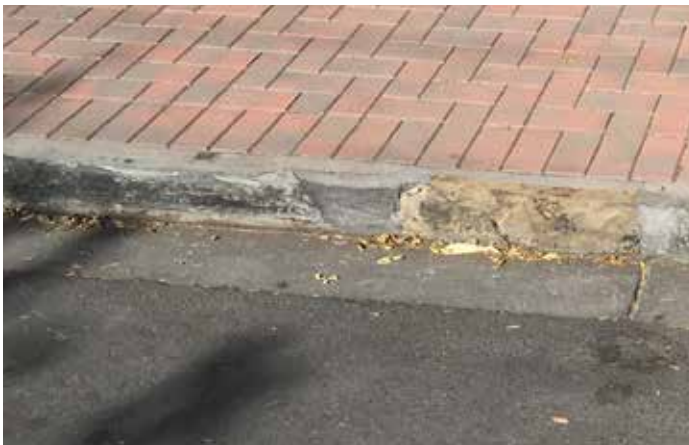
Example stone kerb and concrete water table
