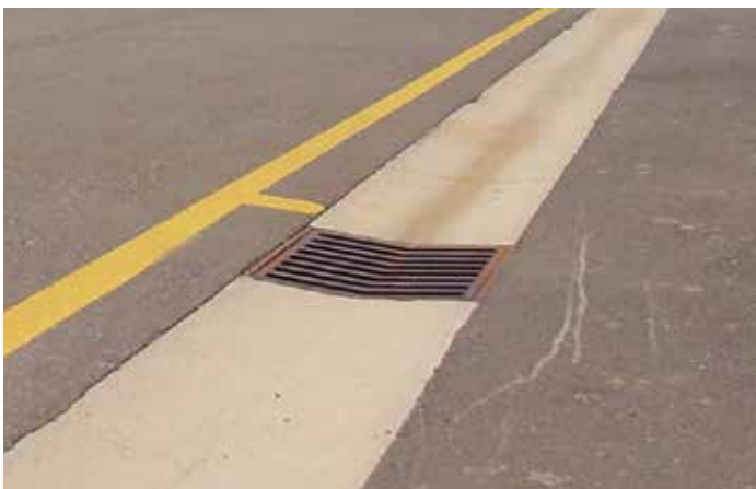
Example concrete spoon drain with grated inlet
