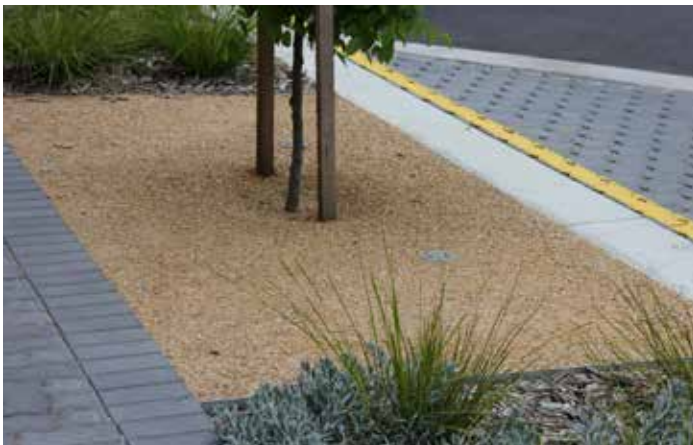
Granulitic sand in verge surrounding tree
