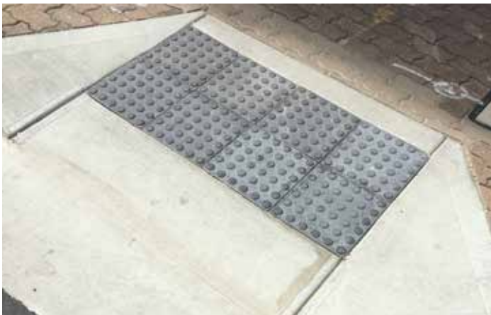
Warning tactiles installed in kerb ramp
