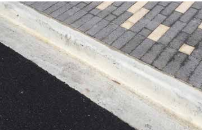
Example concrete kerb and watertable
