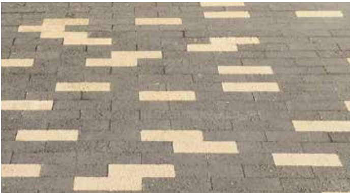
Random colour mix (charcoal 85%, Oyster 15%) in stretcher bond pattern
