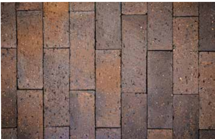
Example pavers (stretcher bond pattern)
